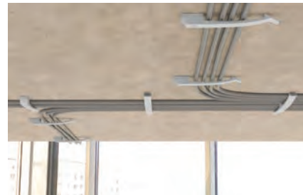
Fixing cable harnesses
