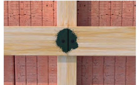
Sealing of the screw heads
