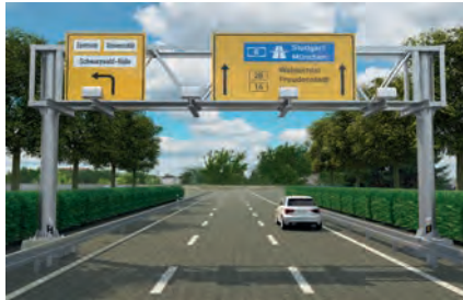
Bridges for traffic signs
