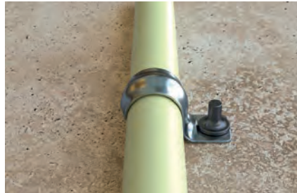
Fixing armoured conduits
