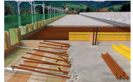
Rebar connections
