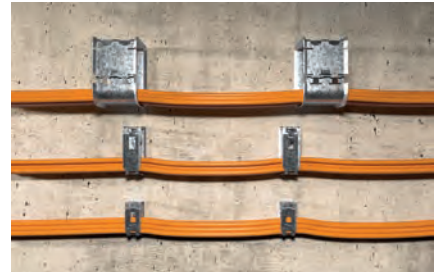
Cable fixing to the wall
