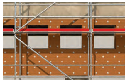
Pressure-resistant insulating materials in curtain façades
