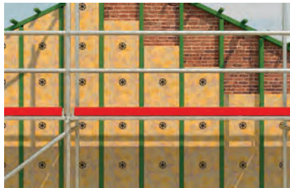
Insulating materials in rear-ventilated façades
