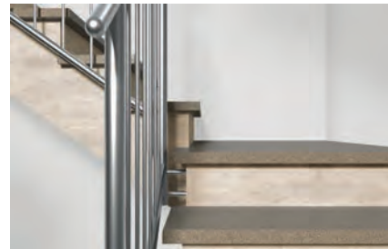
Stair treads on concrete stair stringers
