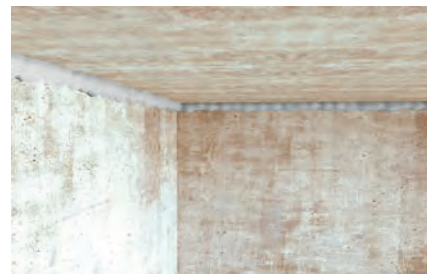
Closing joints in structural work
