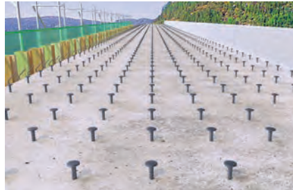
Upgrade of bridges
