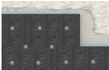
Additional reinforcement of ETICS
