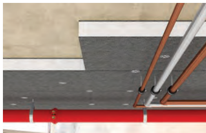
Pressure-resistant insulating materials on ceiling undersides
