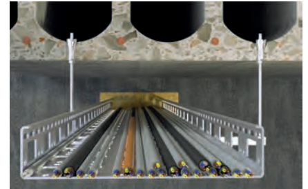
Cable trays in pre-stressed hollow-core concrete
